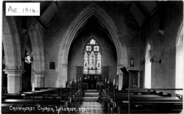
CROWHURST CHURCH, INTERIOR, 1914. The Church showing the Stained Glass Window which was destroyed by a Bomb. Mrs Gibbs was sheltering in the Church at the time.
